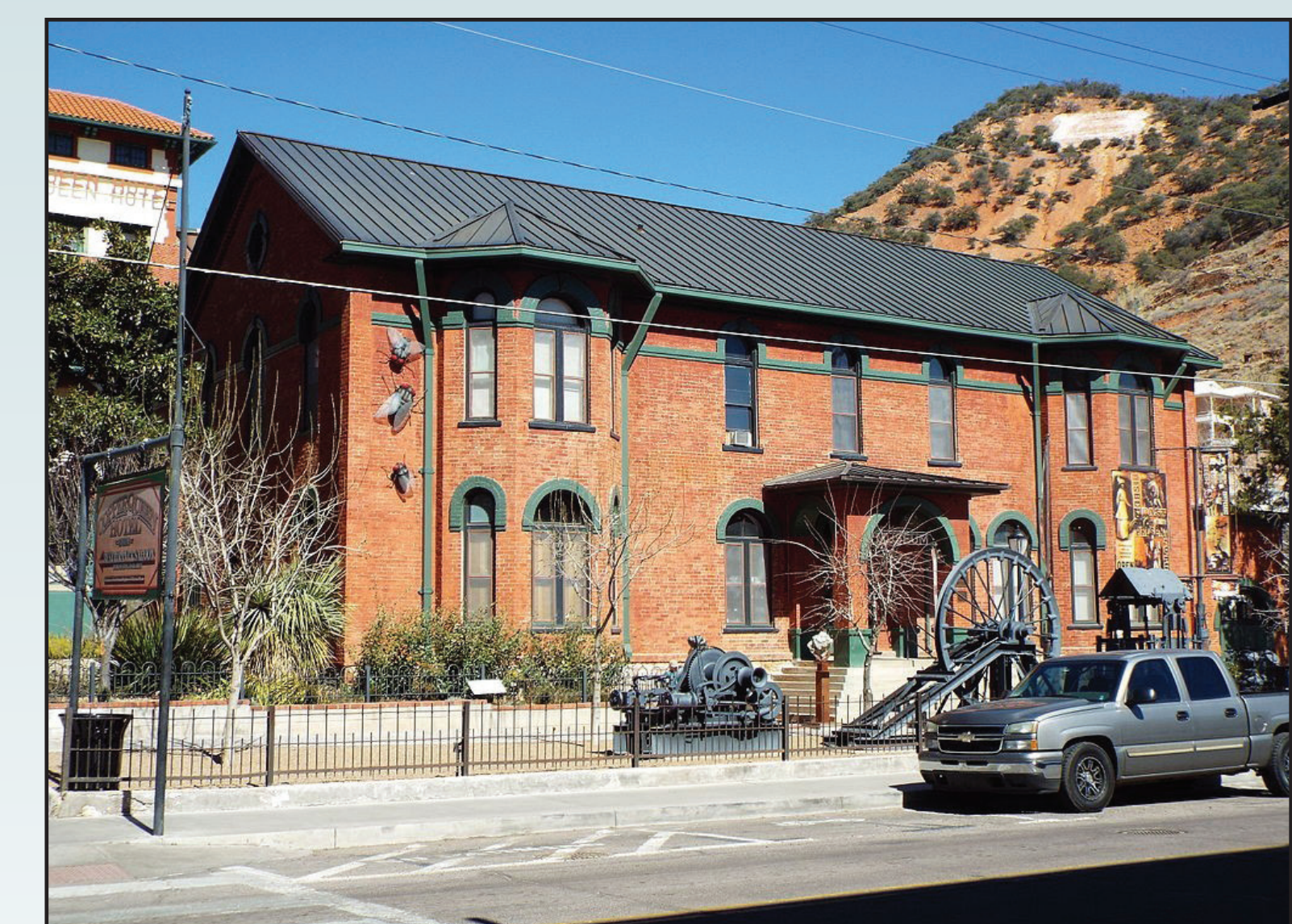
The Phelps Dodge Headquarters Building. (Photograph courtesy Emett, Mike)
